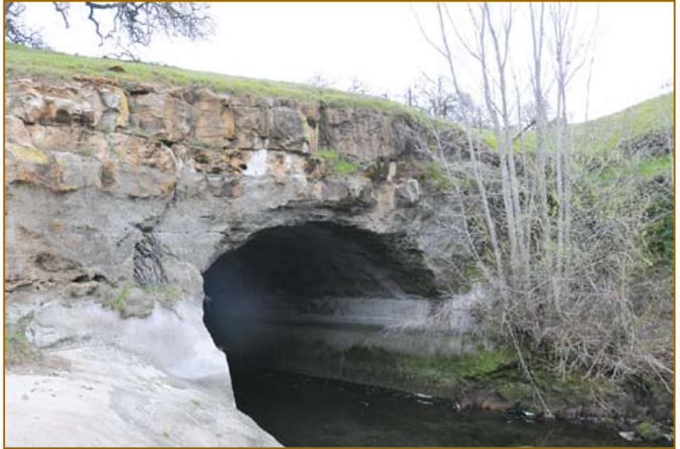
*Tunnel 2 along the Upper Main Canal, seen here, will undergo construction starting this month that involves 'daylighting' the tunnel by transforming it into an open canal.*
